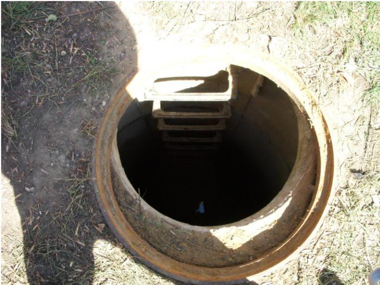
*The incident sewer manhole was five feet in diameter and 18 feet deep with an opening 24 inches in diameter; the access rungs were sturdy and intact (Photo courtesy of NYS DOL-PESH).*
