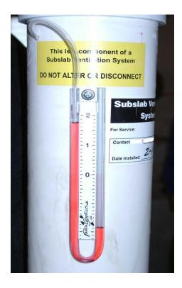
**Figure 5.1** Manometer indicating the SSD system is operating properly.
