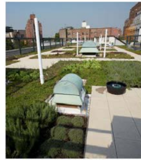
PS 041M with LiveRoof Hybrid Green Roof System (Standard 4.25" Modules and Deep 8" Modules)
