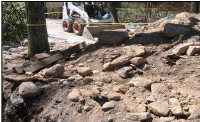
Figure 2: View of the west wall of the excavation south of the “T.” Note the boulders and loose rock/dirt on the excavation face as well as the location of the spoils pile within 2 feet of the edge of the trench. (courtesy of OSHA)
