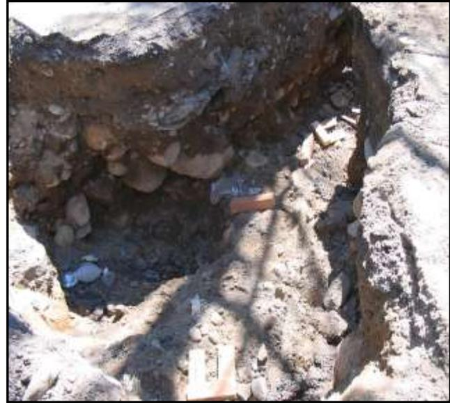
*Figure 4: Area of trench collapse
