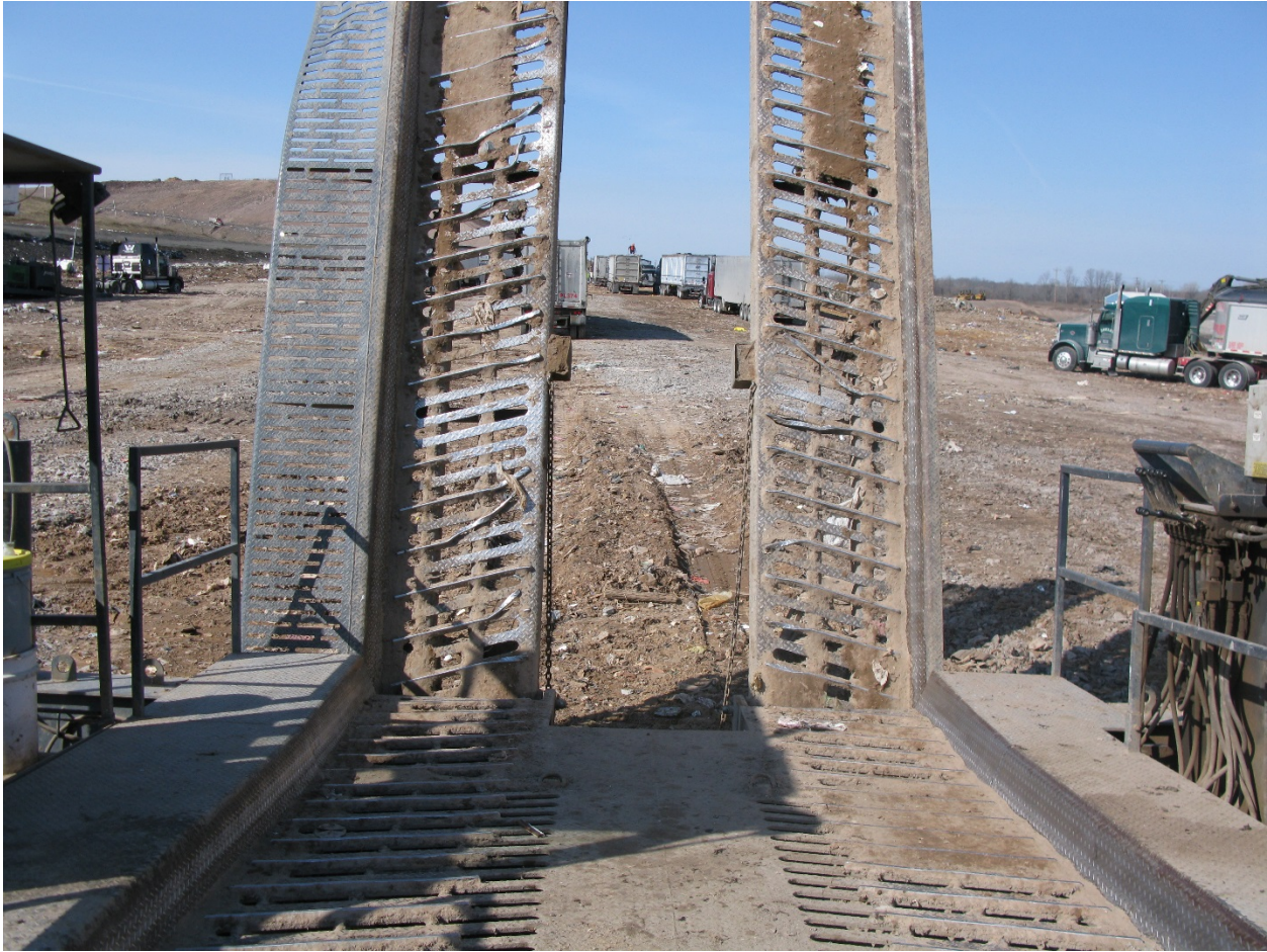
Photo 5. The access ramp is raised to stop the tractor trailer from backing onto the tipper deck when operator is outside the operator's cab.
