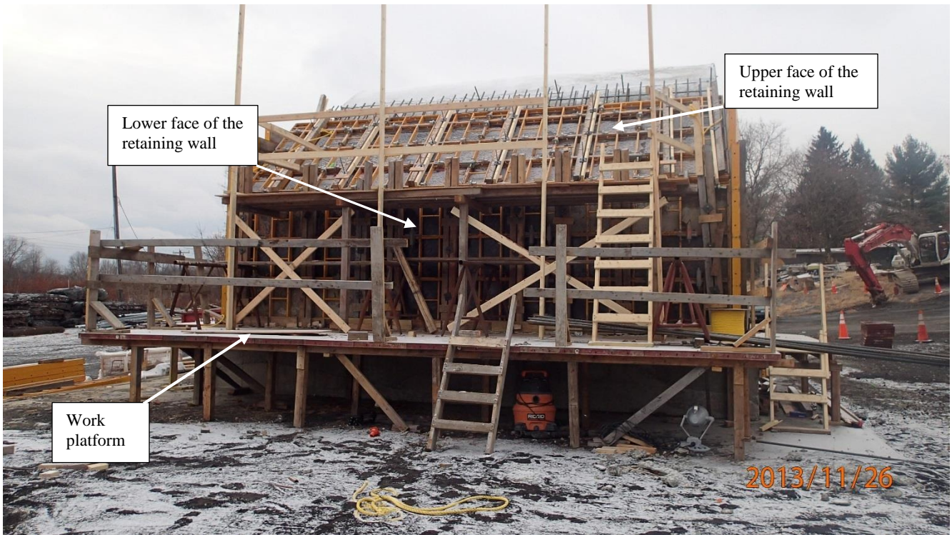
Photo 2. Completed buttress formwork on the morning of the incident.
