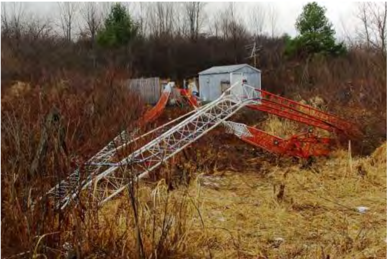
Photo 1. The 380 foot tall guyed tower collapsed killing a 46 year-old tower technician (photo courtesy of OSHA).
